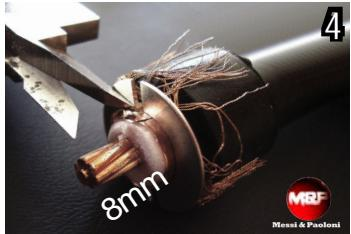
Cut and remove the tape and dielectric for a length as shown in the picture (8mm).
