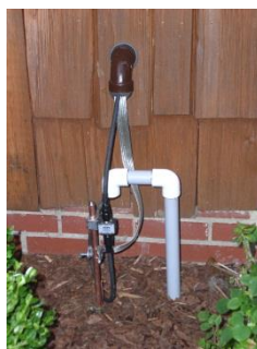
Shack end - Ground Rod and PolyPhaser protection
