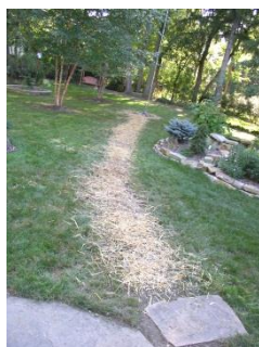
Trench Filled and new grass seeded
